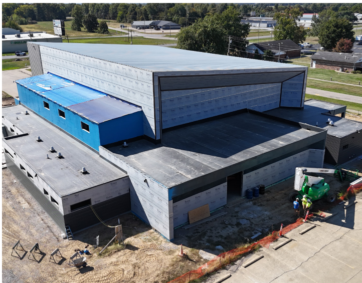
An aerial view of the Jerry Cox Athletic Center on October 7, 2026. Relatively dry weather has helped construction crews make steady progress, with completion expected by December 2026.
