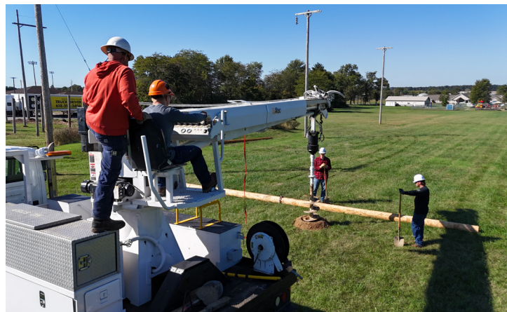
Electrical Distribution Systems Instructor Dustin Wiggins and his students set a southern yellow pine pole using the program's utility truck.
