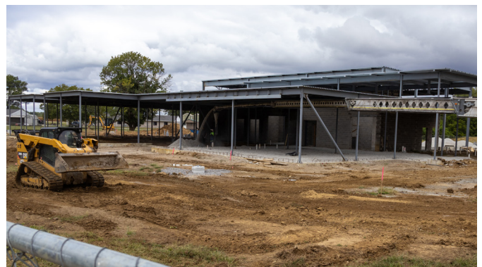
Construction continues on Lincoln Trail College's Career and Technology Training Center, with structural steel and exterior walls taking shape as the project moves toward completion.
