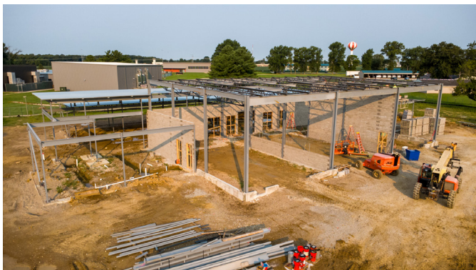
No more imagining where the rooms will be, the walls are going up at LTC's new Career and Technical Training Center!
