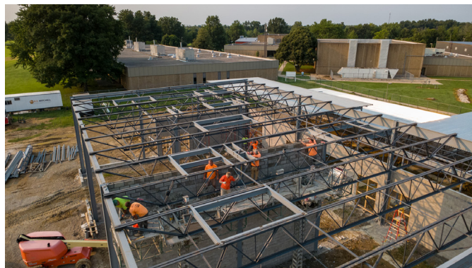
Now we're really raising the roof! Steel trusses are going into place as Lincoln Trail College's Career and Technical Training Center takes shape.
