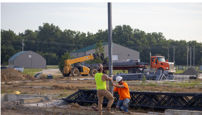
The Technology Center begins rising from the ground as crews guide some of the building's first steel posts into place at Lincoln Trail College.
