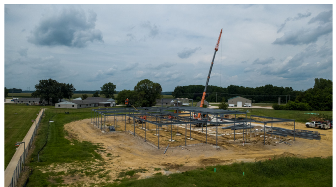
What a difference a day makes! Just over 24 hours after the first steel posts went up, the Technology Center's framework was rapidly taking shape.
