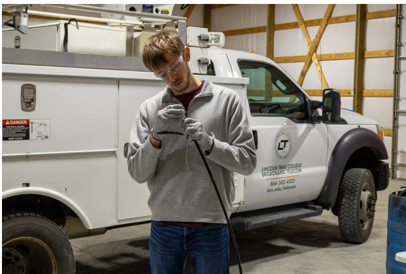
ABOVE: Caleb Gephardt works on stripping a fiber optic cable.
