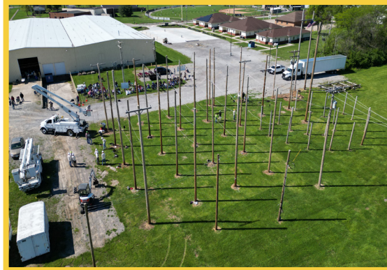
Drone shot of the pole yard
