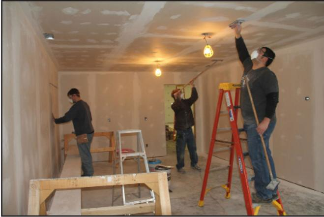
Students enrolled in the Construction Technology Program continue to work at the Wayne County Well Surveys. Most recently they have been installing drywall, mudding the seams, and sanding to a smooth finish. Once the drywall is completed, students will install a ceramic tile floor, and add kitchen cabinets and counter tops.
