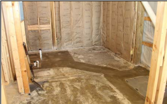
Plumbing has been roughed in and concrete poured in the Bobcat Coffeehouse / student lounge.
