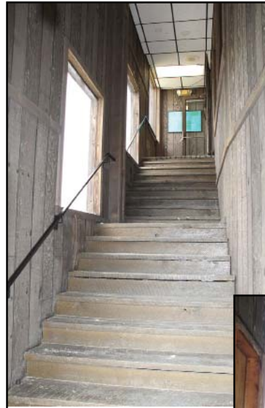
Left: For fire safety purposes, the Construction Tech students cut a door in the top level and built a staircase down to the second level.
