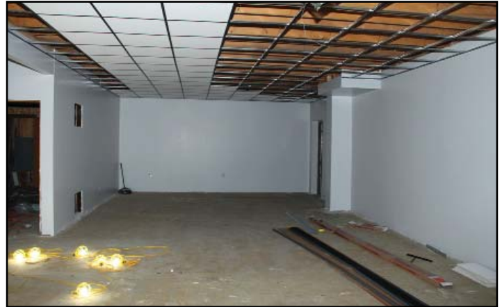
The dry wall is finished and a coat of fresh paint has been applied to the weight room. Ceiling tiles are going in.
