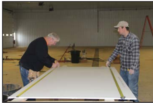
At left, adjunct faculty Larry Barbre discusses the drywall seams with a student. This room will be a restroom.
