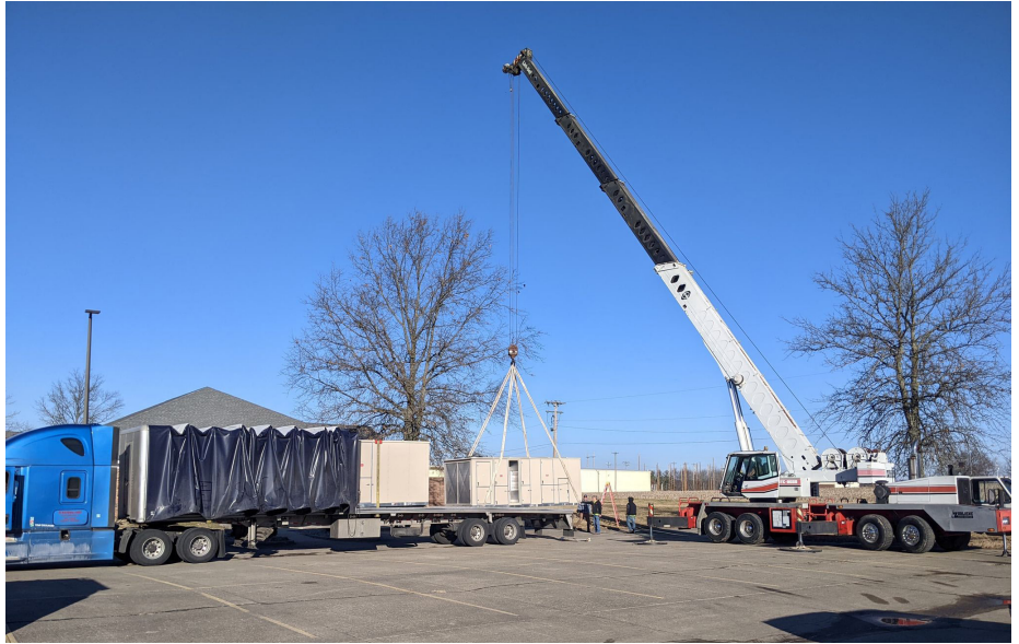
Crane unloading new Mammoth HVAC Unit
