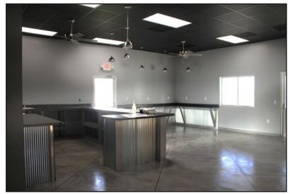
Above: The coffee shop is just about complete. The concrete flooring is finished, the bars, counters, and tops have been installed, as well as the pendant lighting and ceiling fans.
