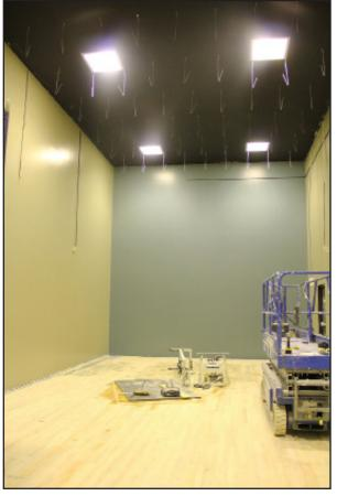
Above: A drop ceiling is being installed in this classroom which will be used for yoga, spin, and zumba classes. Lastly, the wood floor will receive a top coat.
