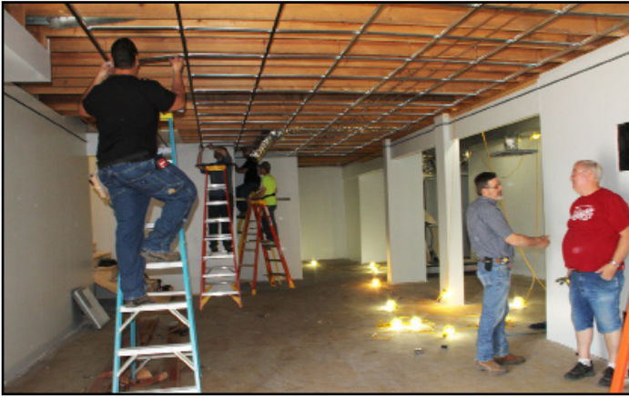
Construction Technology students installed the ceiling grid in the weight room. Adjunct Instructor Larry Barbre shown at right in blue shirt is overseeing the students' work.
